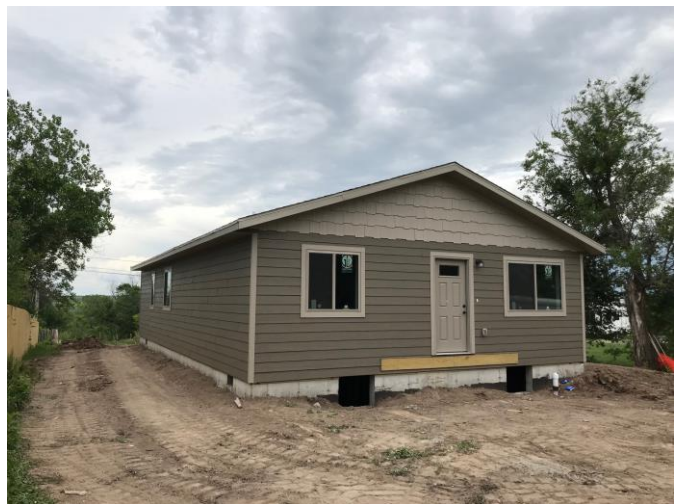
Getting ready for finishing touches.
