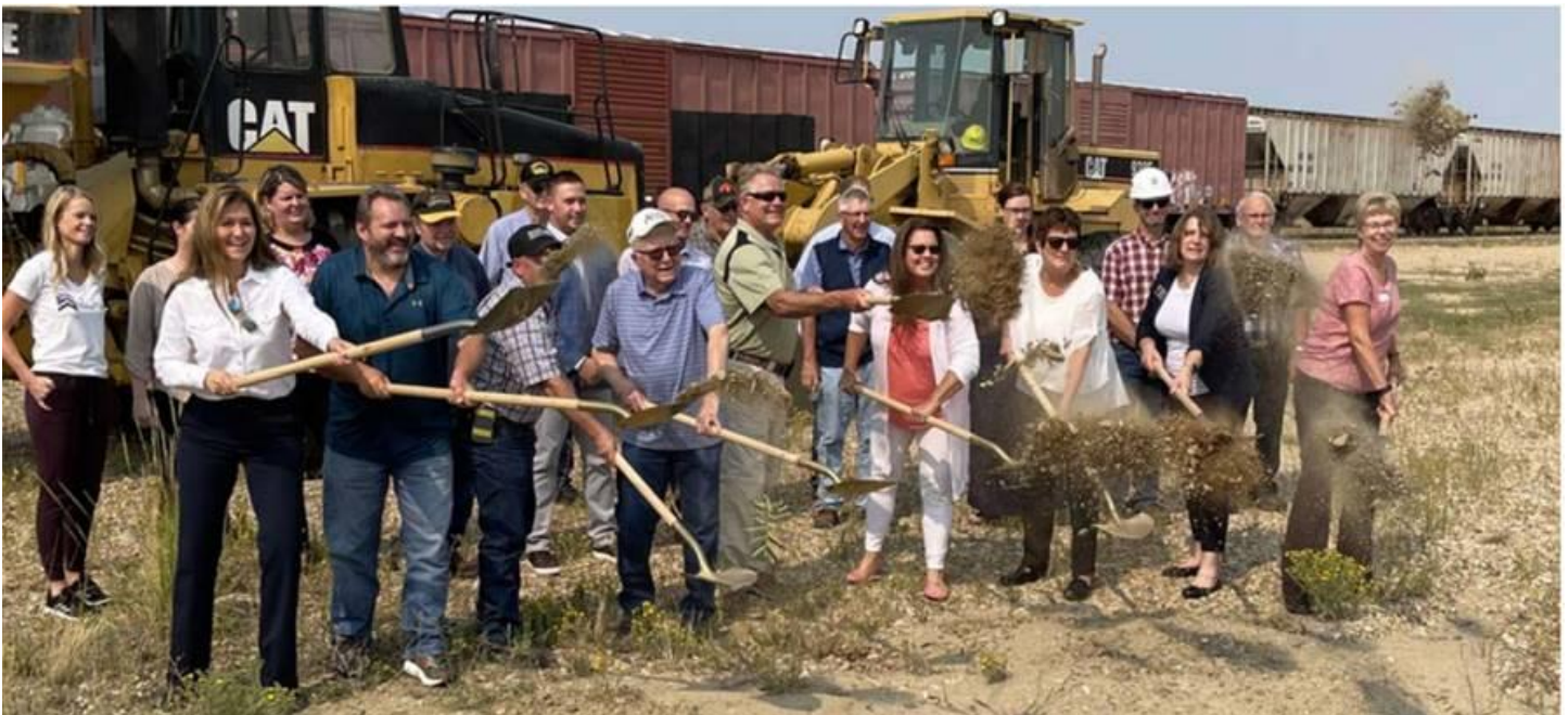
Hollie Stalder leads a group of representatives from several local and state organizations in tossing the first shovelfuls of dirt into the air at the ground breaking for the Industrial and Rail Park’s long-awaited rail siding expansion project. Front row - left to right: Hollie Stalder, Executive Director Belle Fourche Economic Development; Jeff Burket, South Dakota Railroad Board; Randy Schmidt, Belle Fourche Mayor; Stan Harms, Butte County Railroad Authority Chair; Greg Car, South Dakota Railroad Board; Karoll Herman, Butte County Commission Chair; Karen Wagner, Belle Fourche Economic Development Industrial & Rail Park Committee Chair; Lori Frederick, Governor’s Office of Economic Development; Renae Schaeffer, Belle Fourche Economic Development President. - Beacon Photo
