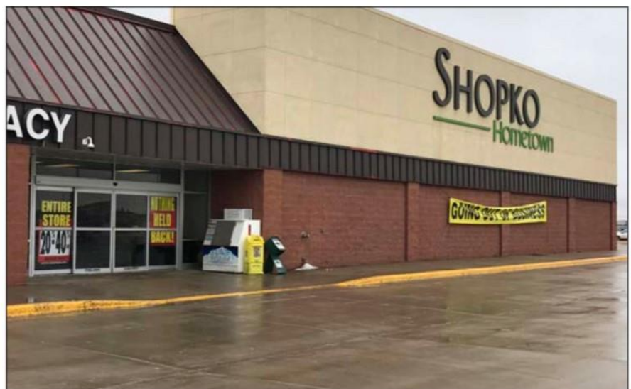
FIREFLY BUILDERS, INC WILL MOVE FROM THEIR CURRENT OFFICE AT 1411 5TH AVENUE TO THE OLD SHOPKO BUILDING. -BEACON PHOTO
